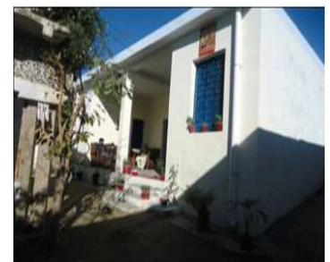
A View of Newly Constructed House in Charsadda
