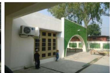
Basic Health Unit After Repair
